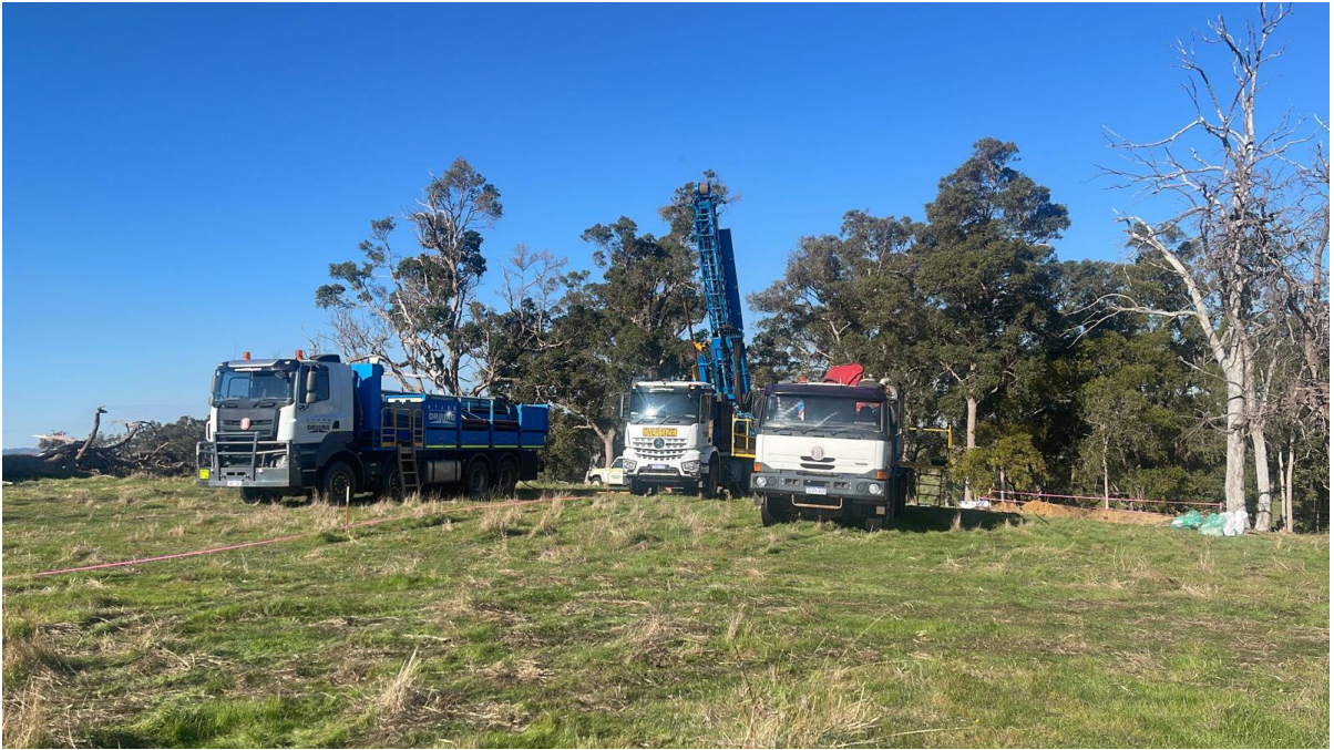
Figure 2: Drilling in an open paddock
